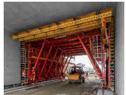
In accordance with the occurring loads, it is possible to realise supporting structures with diagonal struts or trusses with the Vertical Post.
