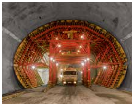
For mined tunnels, access portals are an important prerequisite for use.
