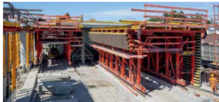
Smart engineering solutions with a folding mechanism allow PERI UP back-propping, resulting in early moving of the formwork carriage.
